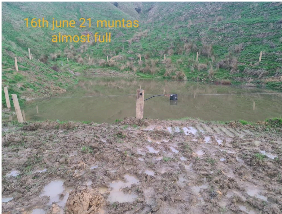
Figure 6: New sediment trap on Nelson's filling up.
