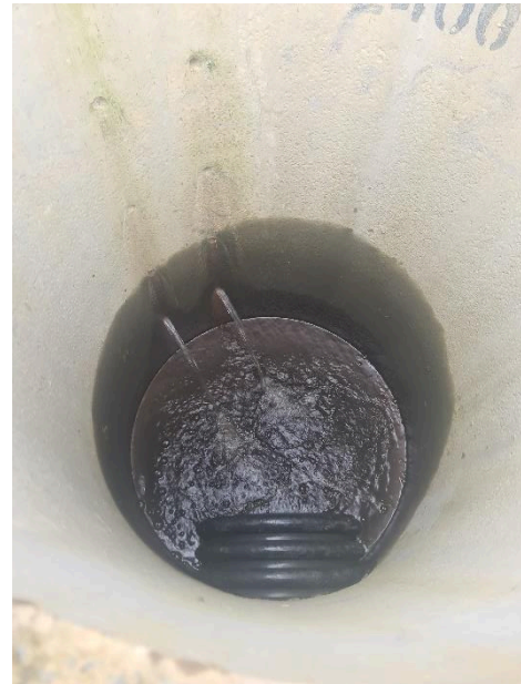
Figure 9: Flow through the riser system
