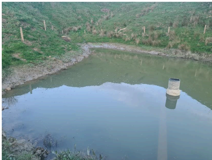
Figure 29: Sediment trap for 3.6 ha catchment
