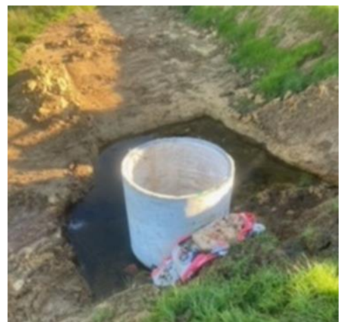
Figure 12: Proffit riser at installation
