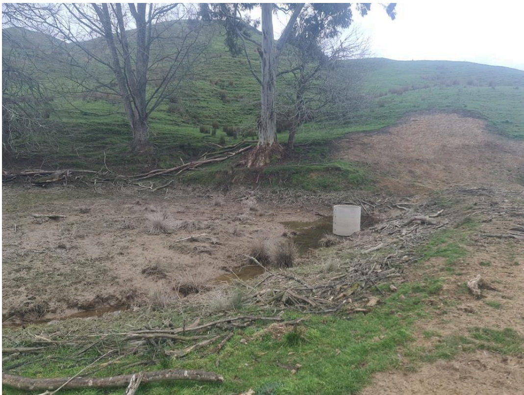
Figure 10: Foss site after it has slowly emptied through the riser pipe system
