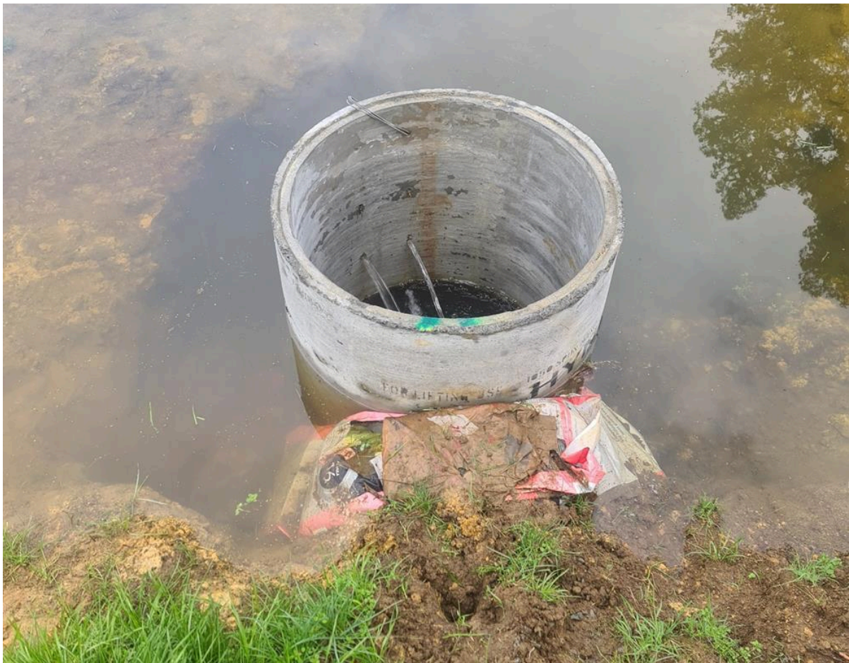
Figure 13: Water flowing into the riser pipe slowly as the water level increases
