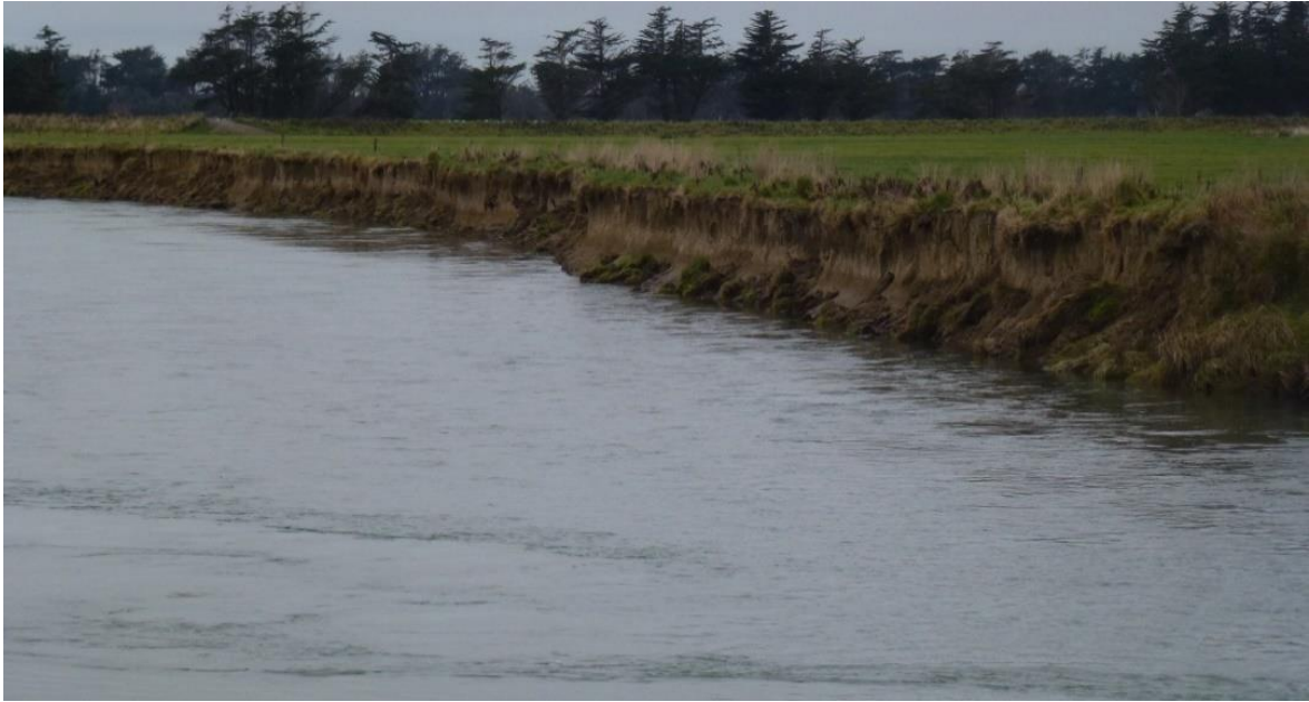
Figure 9. Bank erosion in the lower reaches of the Oreti River, June 2018. Note the stopbank in the front of the trees.
