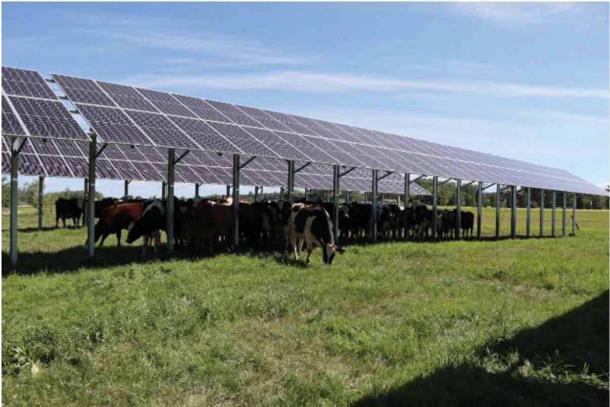
Figure 10. Single pile system at the University of Minnesota West Central Research Outreach Centre (WCROC).
