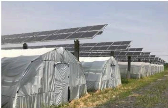
Figure 36: PV modules over a foil tunnel. © BayWa r.e.
